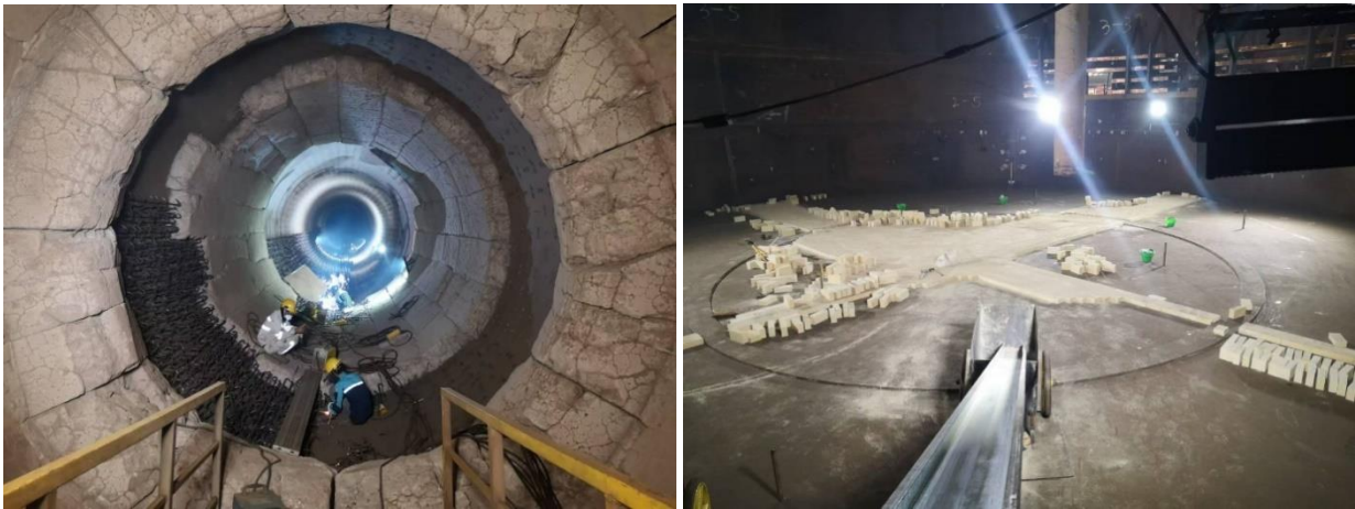
Figure 4: BSI RKEF furnace refractory relining
