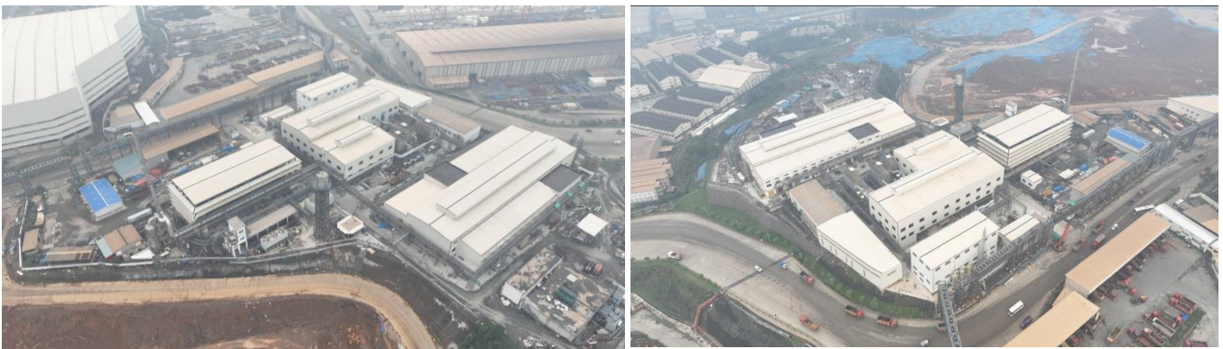
Figure 17: Construction of CCP
