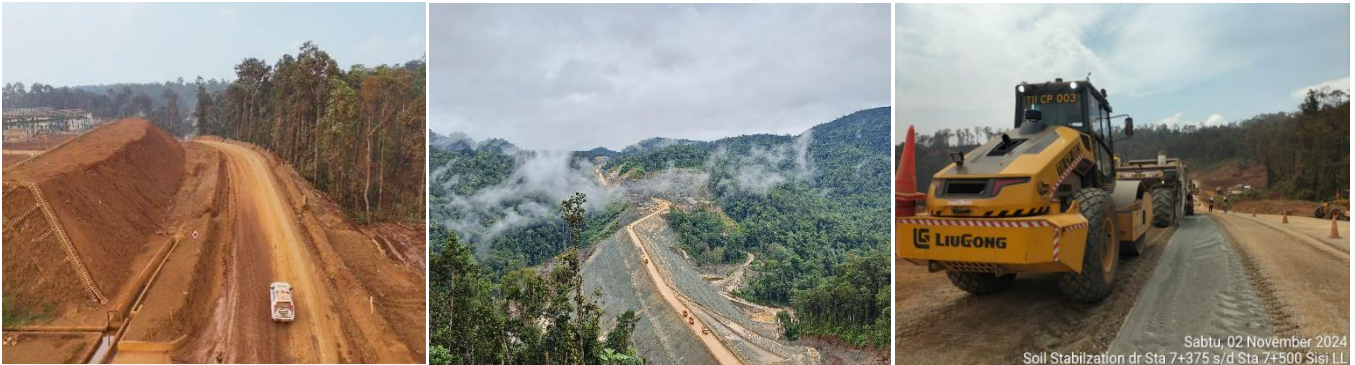
Figure 3: Mine roads (left and centre photo); Road improvement works (right photo)
