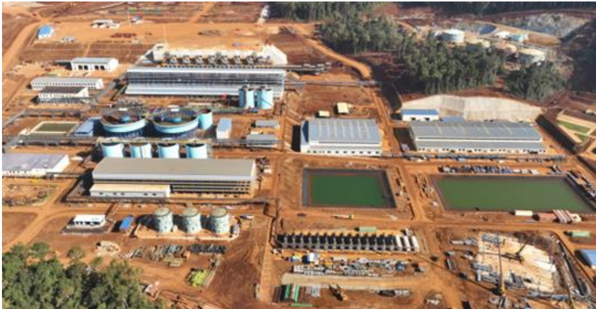
Figure 5: FPP at the SCM Mine concession area
