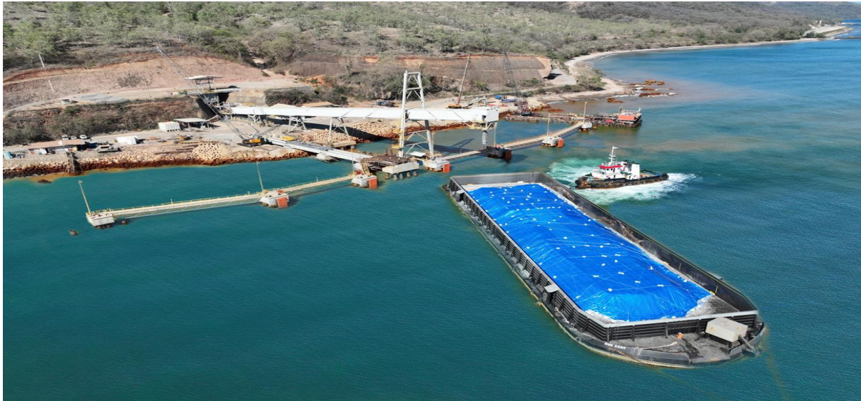
Figure 11: Wetar barge jetty
