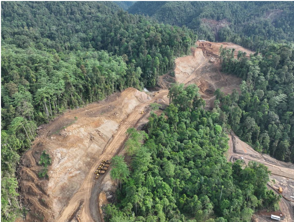
Figure 1: New haul road construction progress
