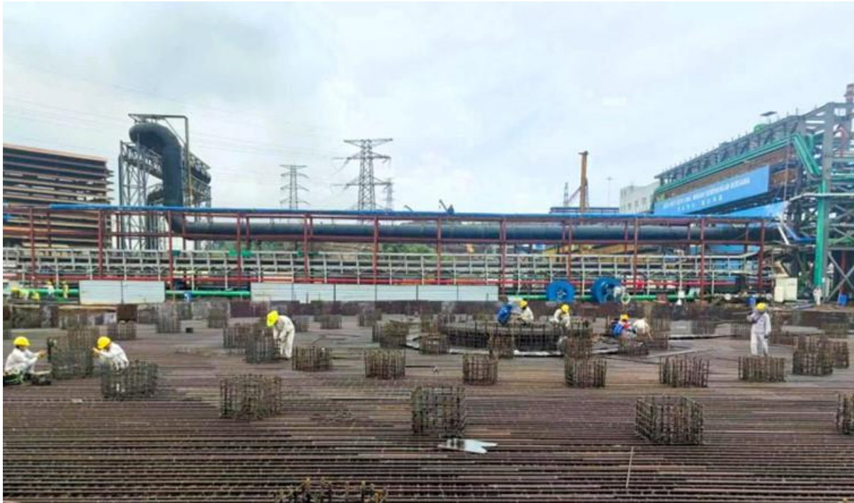
Figure 4: PT ESG HPAL foundation work
