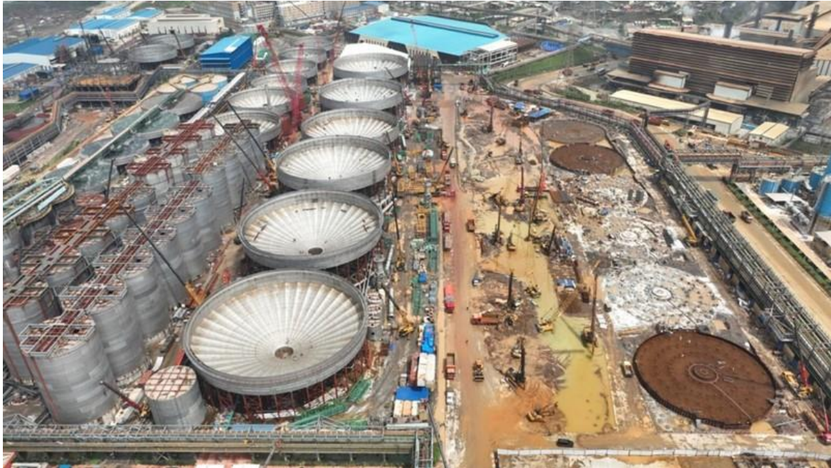
Figure 6: PT ESG HPAL plant construction progress
