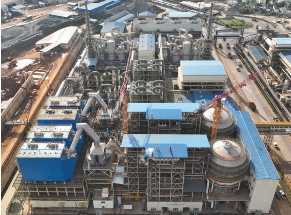
Figure 3: AIM acid plant
