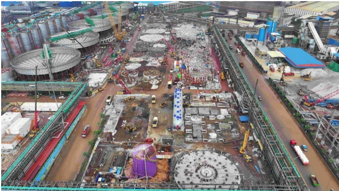
Figure 4: PT ESG HPAL plant construction progress
