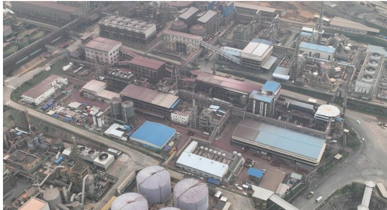
Figure 16: Chloride plant operations
