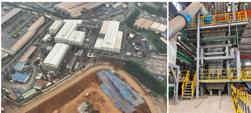
Figure 17: From left to right: 1) Copper Cathode Plant; 2) Blast Furnace
