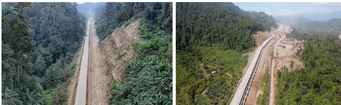
Figure 3: Slurry pipelines construction parallel to hauling roads (left); Hauling roads extension (right)
