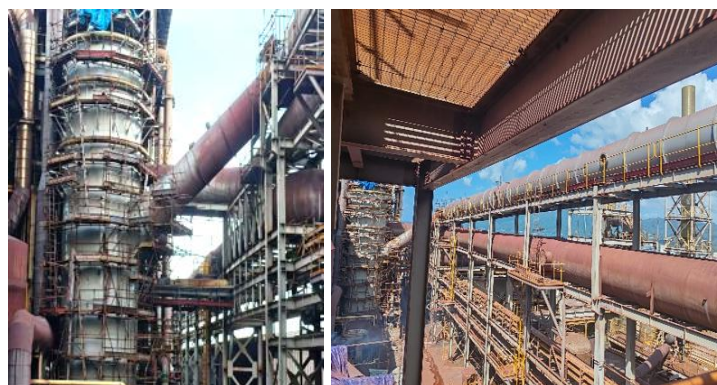
Figure 16: Chloride Plant – New Cooling Tower and Flue Gas Pipeline
