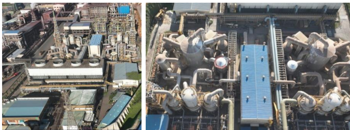
Figure 15: Acid Plant operation
