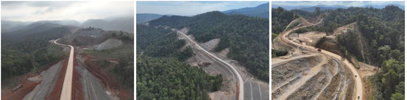
Figure 3: Mine roads extension (left and centre photo); Mine roads widening (right photo)
