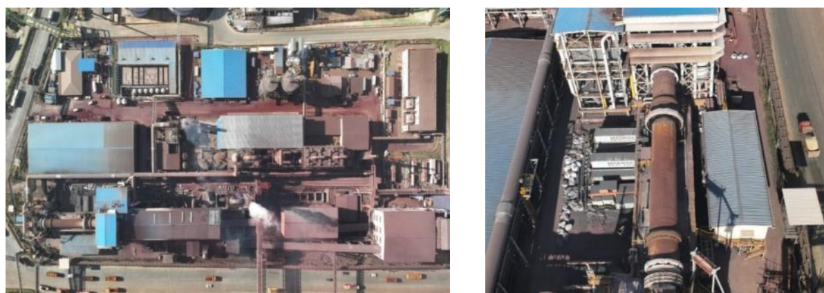
Figure 16: Chloride plant operations
