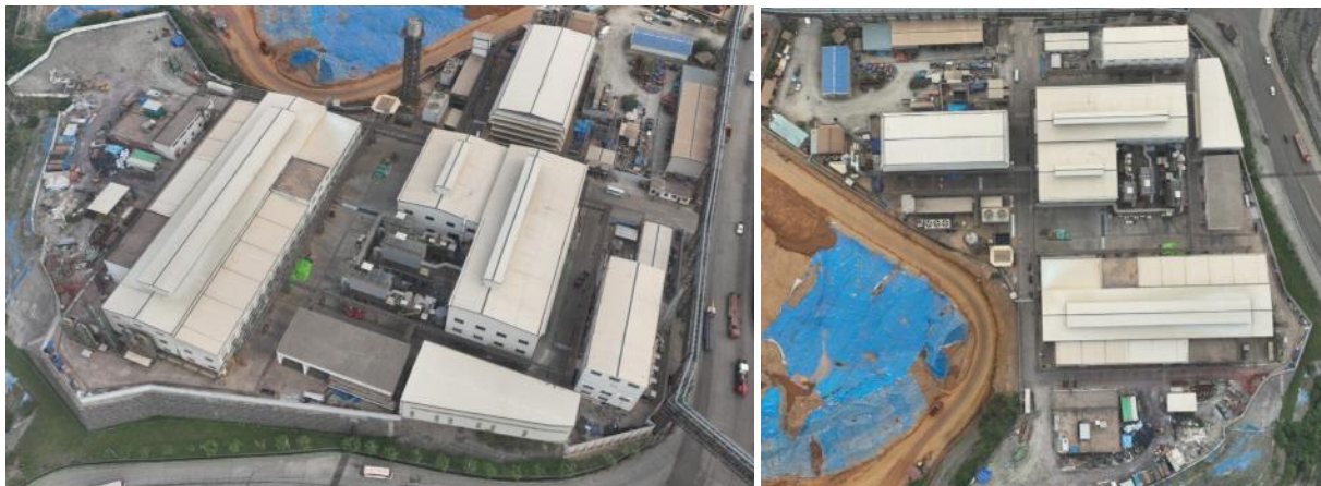
Figure 17: Copper Cathode Plant
