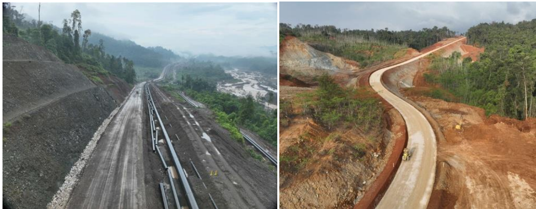
Figure 3: Slurry pipelines construction parallel to hauling roads (left); Hauling roads extension (right)
