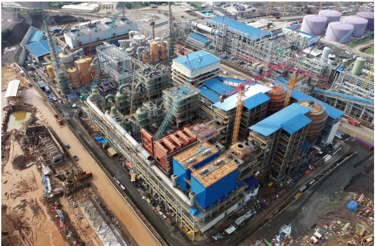
Figure 7: Construction progress of AIM Project
